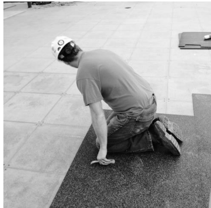
Square Cut Glue Down Installation
